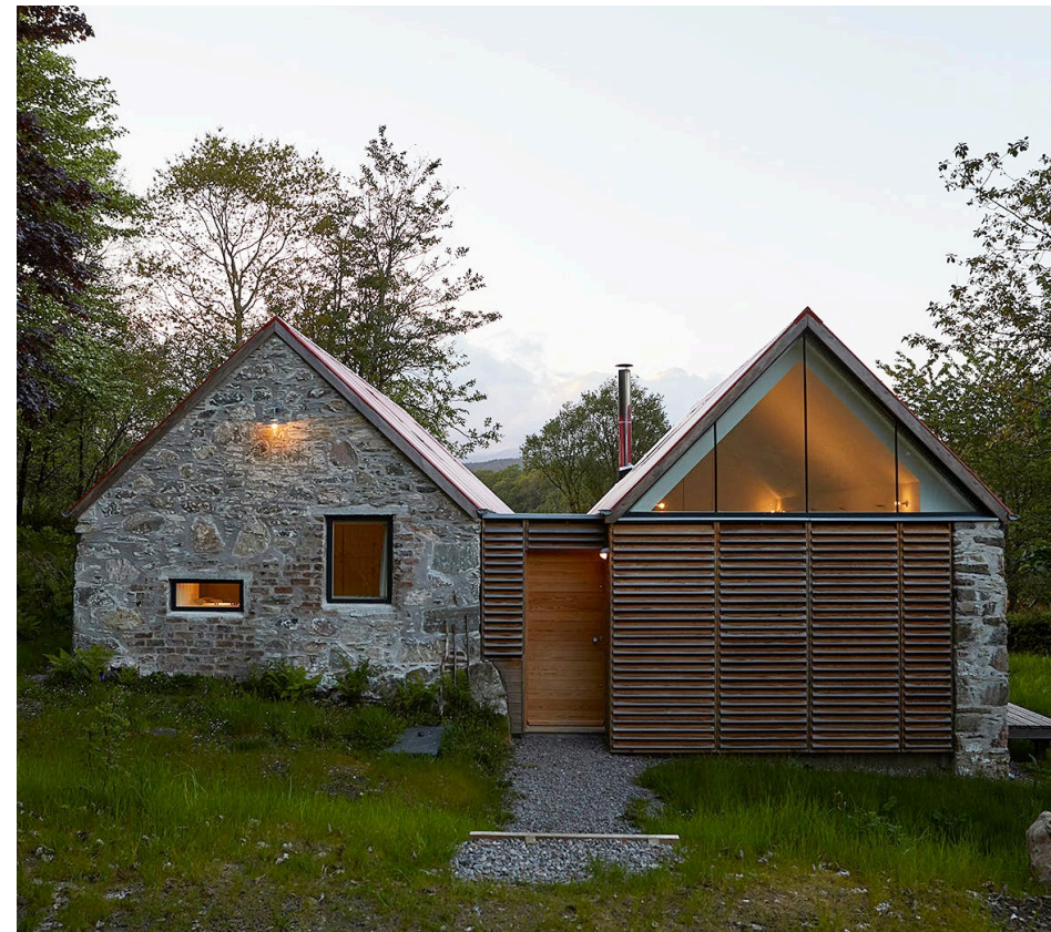
Stone and timber precedent building
